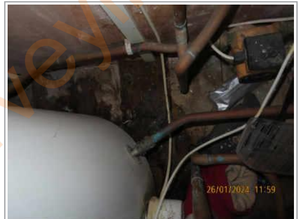
Leak on cylinder
